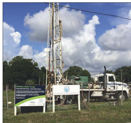
Figure 6. The first of three cores associated with TAP Alternative 2 is almost complete.
